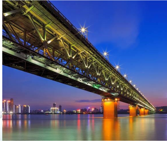
Structural health monitoring
