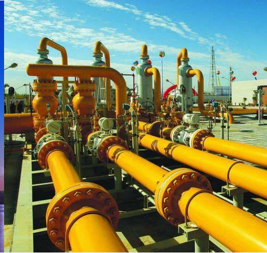
Pipeline leakage detection
